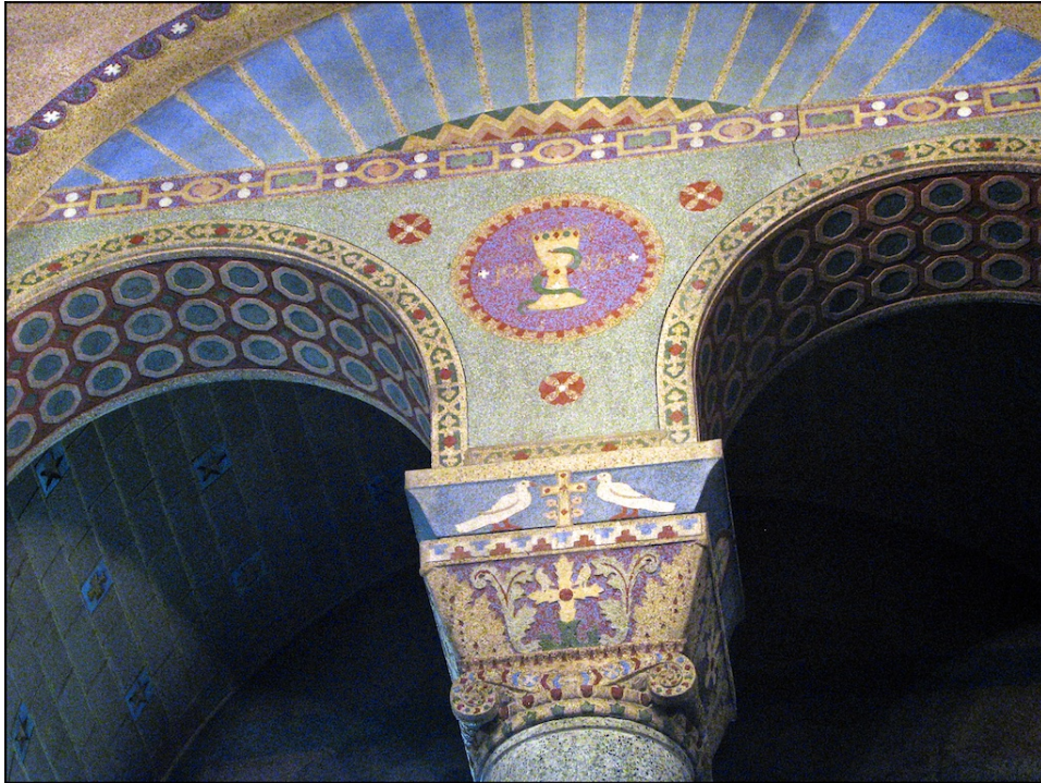
Figure 1 John Earley stunned the industry in 1921 by creating breathtaking colors, forms and textures with exposed aggregate polychrome mosaic concrete for the interior of the Shrine of the Sacred Heart.
