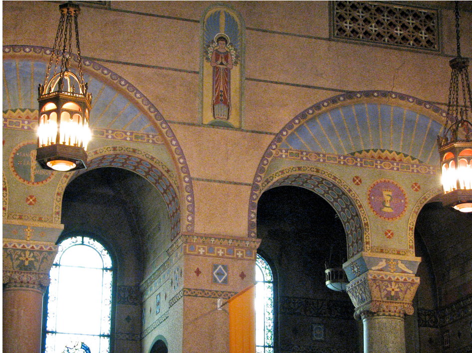
Figure 3 — For architectural decoration and moldings, Earley Studio installed polychrome mosaic concrete as thin, precast slabs and applied stucco with great precision.
