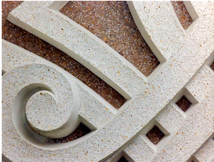
Figure 7 — Polychrome mosaic concrete panels for the Baha'i Temple display remarkable precision in delineation of the color, sharp arrises, uniform exposure of the aggregate and a third chroma effect by not exposing the sides.
