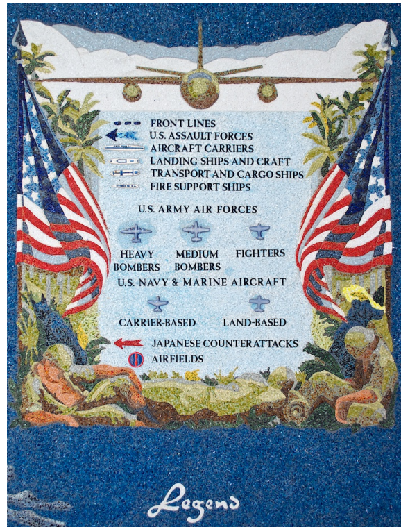
Figure 9 — This 18 in. (450 mm) by 24 in. (600 mm) legend on the battle map includes plastic letters and glazed ceramic symbols among flags, soldiers, plants, an airplane and clouds created with polychrome mosaic concrete.
