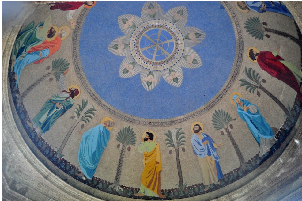
Figure 5 — Thin, precast slabs were prepared on curved molds in the studio for the figures and decoration. The thin, precut slabs were installed on the dome with a brown coat before mosaic stucco was applied around
