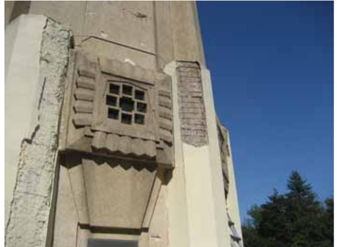
**Field investigations at the Edison Memorial Tower revealed a range of deterioration caused by two factors: corrosion of the embedded reinforcing steel and cycles of freezing and thawing** (Photo courtesy of Mills + Schnoering Architects, LLC)
