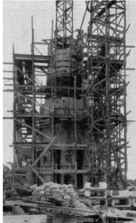
Earley's last major project, the Edison Memorial Tower, was created with a sophisticated blend of concrete aggregates.<sup>8</sup> The precast concrete panels feature a sequence of color gradations: the darkest color is at the bottom and the lightest is at the top
