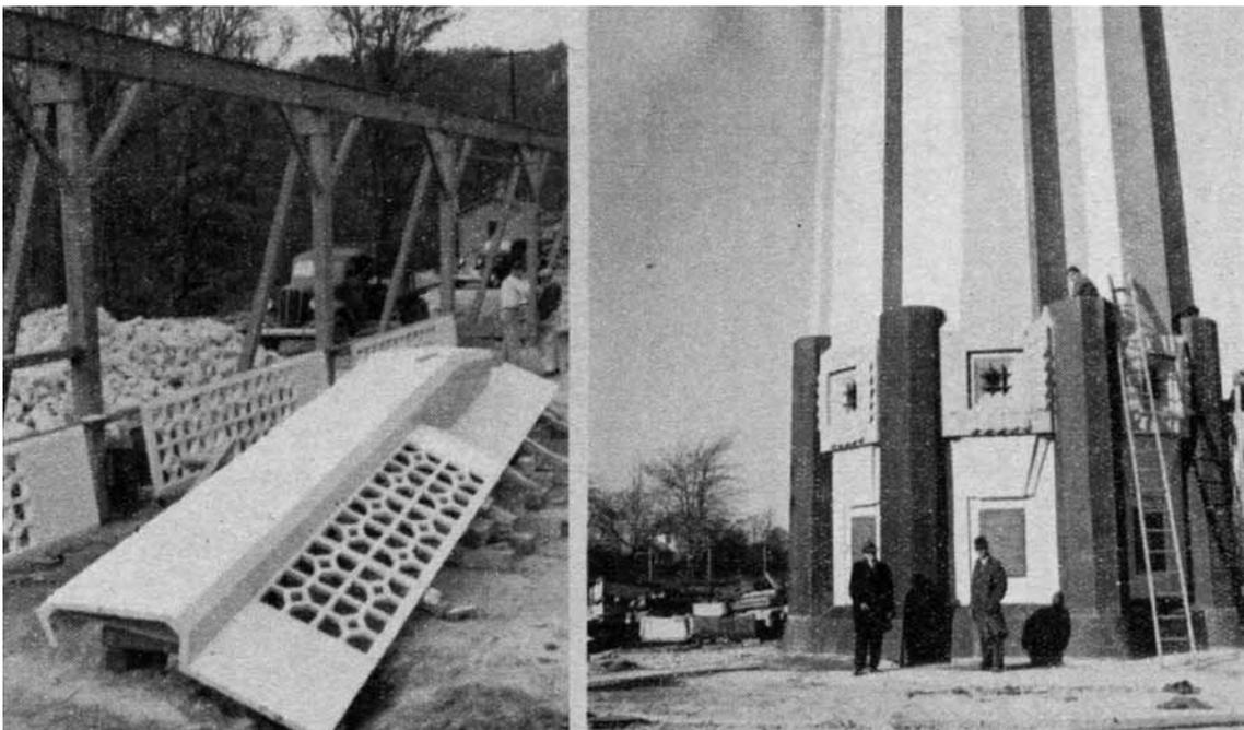
The panels for the Edison Memorial Tower were precast in Earley's studio in Virginia and shipped to the site in New Jersey.<sup>8</sup> Concrete grillages were installed over the loudspeakers at the top and bottom of the tower
