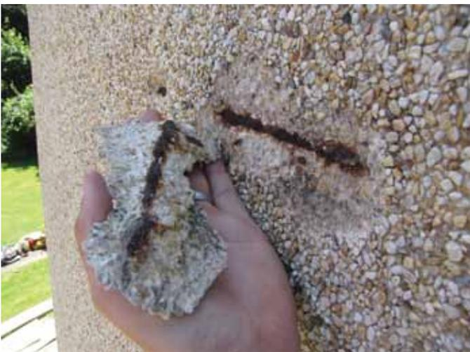
**A corroded reinforcing bar behind the exposed aggregate concrete facing of the Edison Memorial Tower** (Photo courtesy of Mills + Schnoering Architects, LLC)
