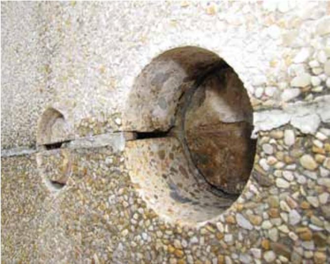
Concrete cores were taken from the Edison Monument to allow for laboratory analysis of the panel concrete. Panels were composed of a face mixture and a backup mixture. The panels served as the exterior forms for reinforced concrete that provides structural support of the monument (Photo courtesy of Mills + Schnoering Architects, LLC)
