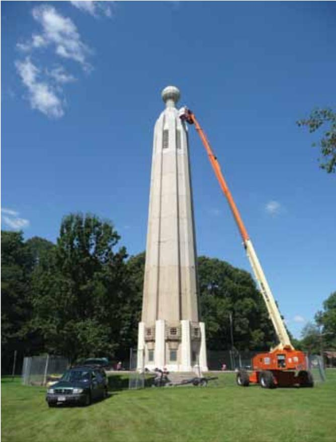
With its concrete heavily deteriorating, the state of New Jersey hired Mills + Schnoering Architects, LLC, to restore the Edison Tower. Field investigations in 2009 revealed that some panels, mostly the ones at the top, had to be completely replaced (Photo courtesy of Mills + Schnoering Architects, LLC)
